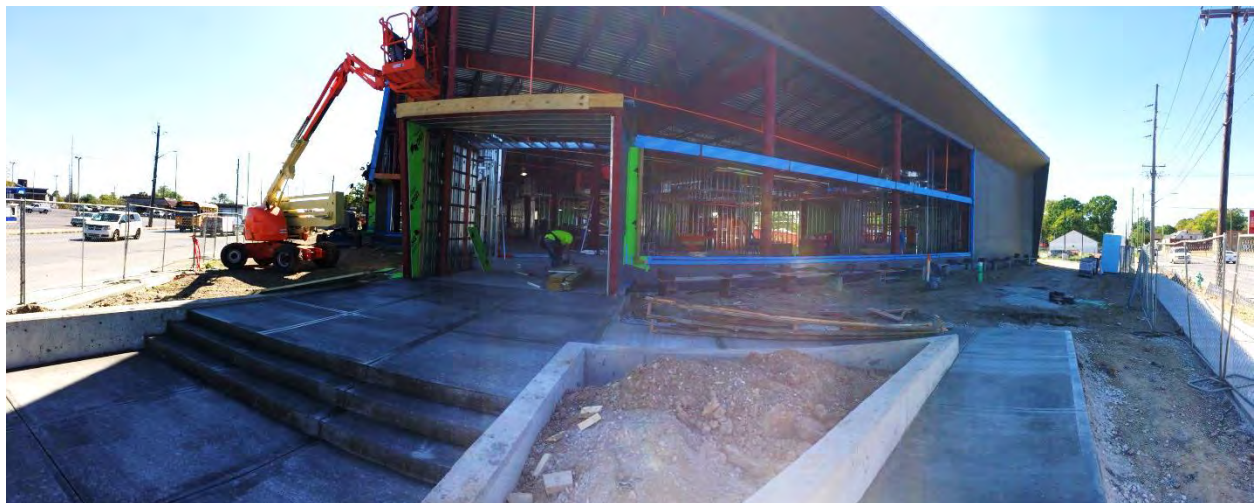
Project Site on October 10, 2019 Exterior panoramic view of the Sherman Entrance.
