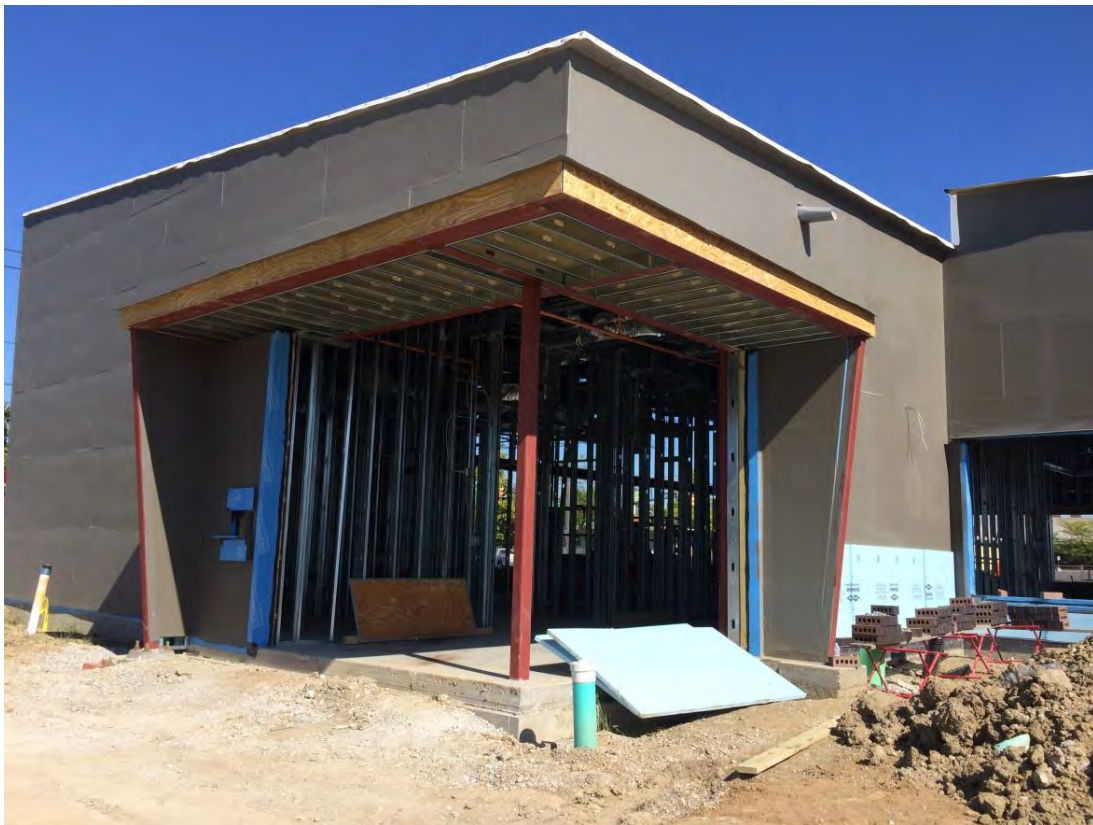
Project Site on October 10, 2019 Exterior view of the West Entrance.
